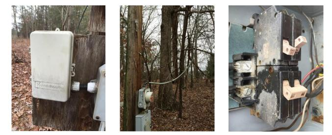
Enter Chuck Dyba and his team at Unlimited Electrical Contracting (formerly Gaddy Electric in Goode). A new pole, service wire, meter base, breaker box, and junction housing were installed providing a thorough and safe upgrade of electrical service.
