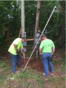
None of this would pass code. So at this point it was decided that there was no choice but to replace everything. This involved boring under both roadways and the median "island" and putting in a flexible conduit into which new wires will be run to the walls and the gazebo.
