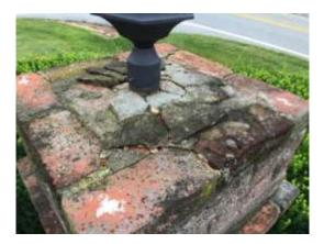
Further examination revealed that several bricks and mortar were loose on three of the pillars and that the cement cap needed to be replaced on all six pillars.
