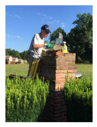
Once the loose bricks and mortar had been removed, the re-building process proceeded smoothly.
