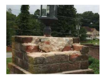
Some of the pillars were in such poor condition that several courses of loose brick and mortar had to be removed.
